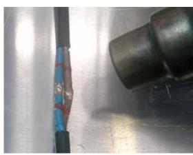
8. Slide the heat-shrink tube over the joint, ensuring that the heat-shrink tube covers each end of the joint evenly and start to heat the tubing from the centre outwards.
